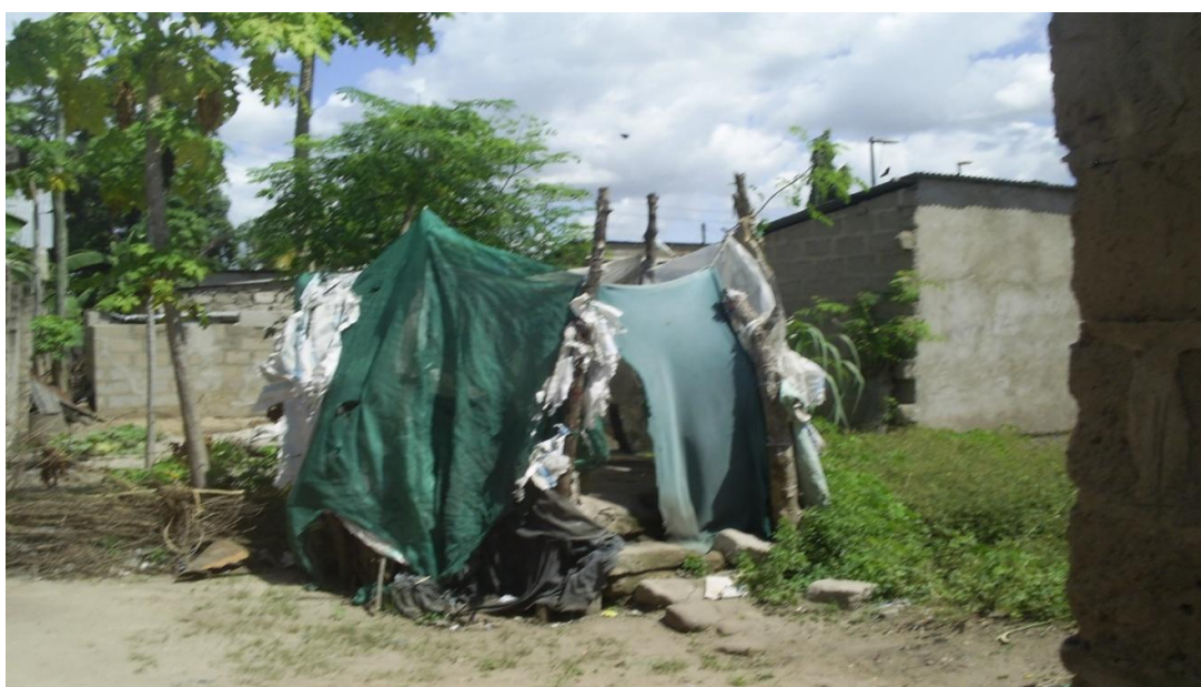
Figure 1: A picture showing residential buildings and type of toilet in Makangarawe
